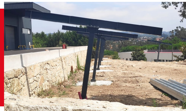
Steel pipe beams PRS200X15 + 250X8 + 100X15mm S275JR
